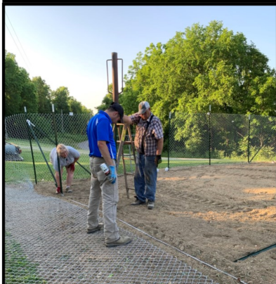
Fencing going up at High Hill Presbyterian Church Garden.
